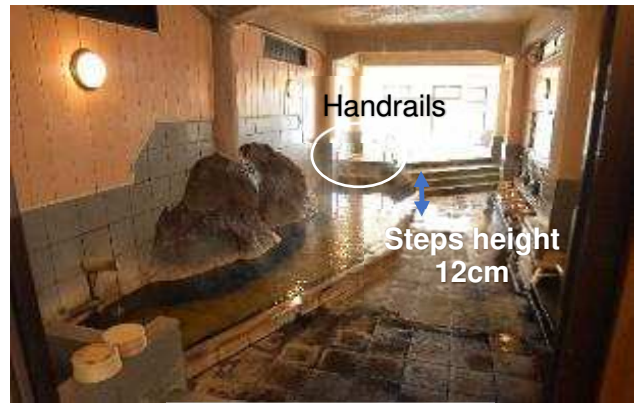
Communal bathhouse There are steps inside the bathtub Handrails Steps height 12cm
