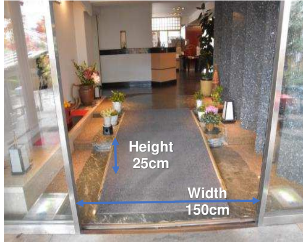
Slope to the entrance
