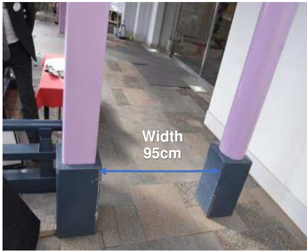
Slope to the entrance
